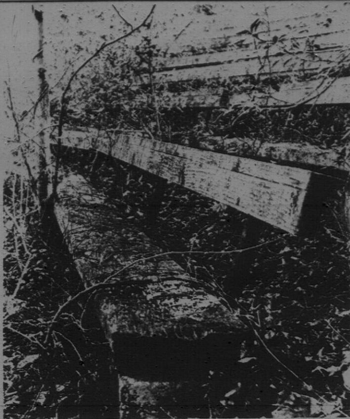
Nearly forgotten now, the theatre quietly decays.
