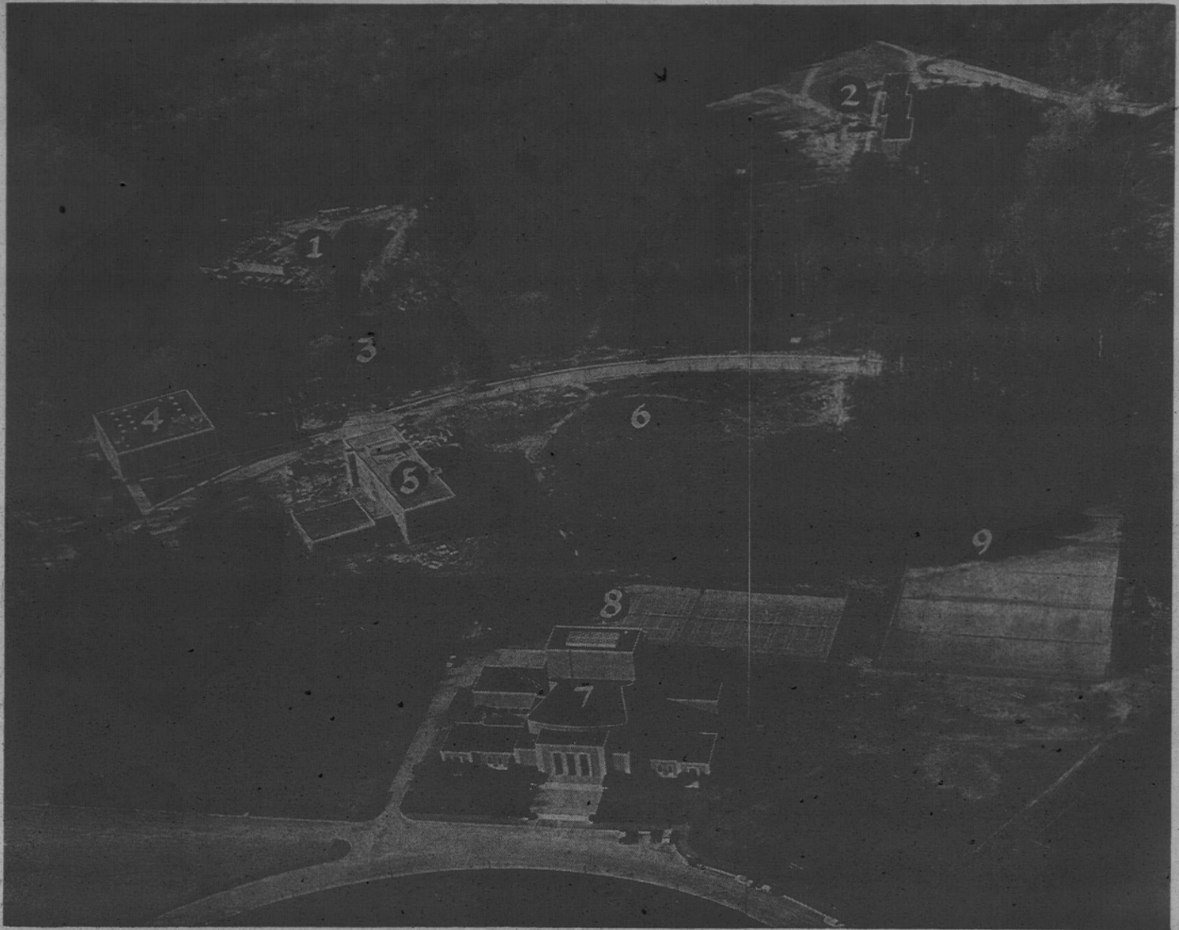
NEW CAMPUS — 'CENTER OF ADVANCED ARTS AND SCIENCES' CONTINUES TO GROW
