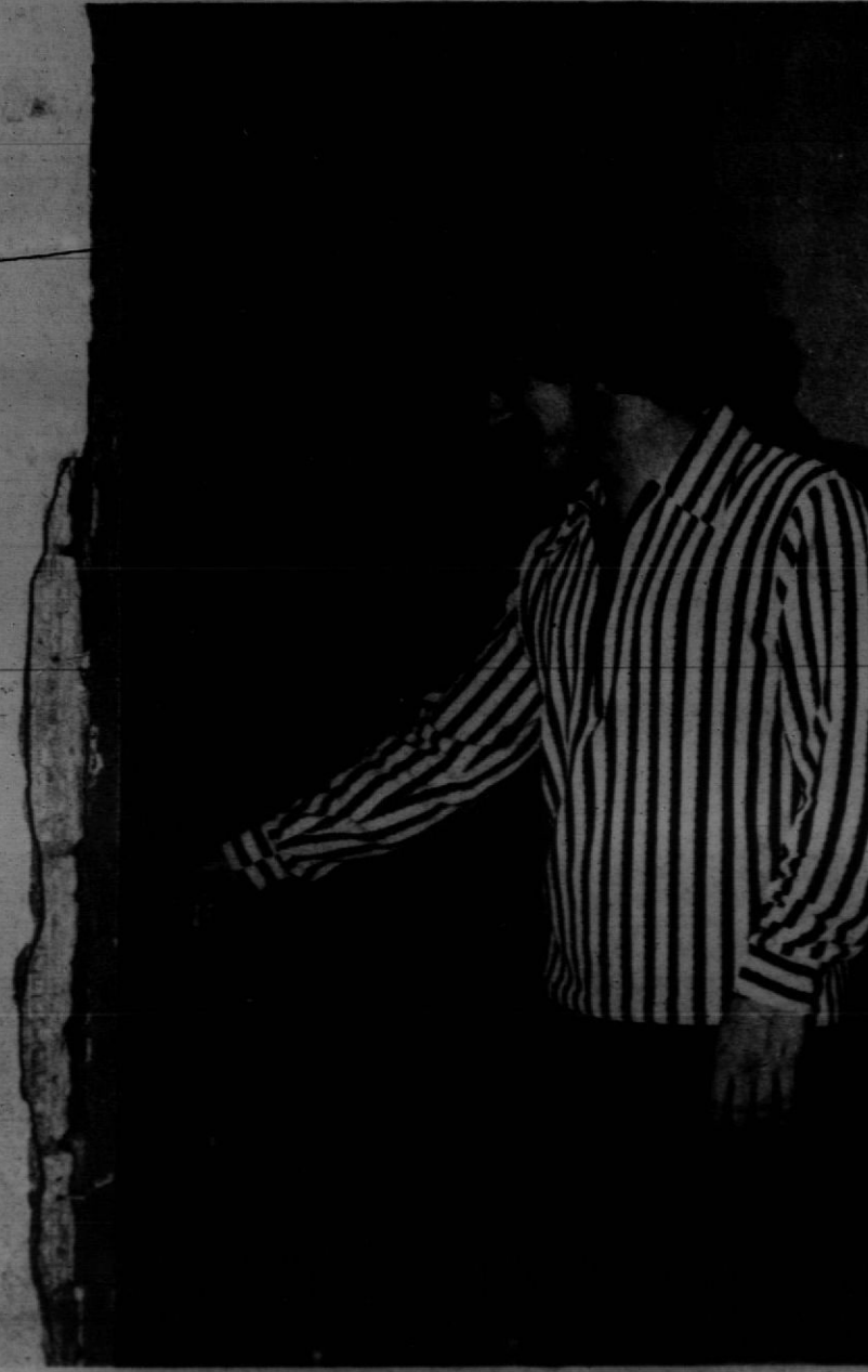
Missing plaster by Bullock's door
