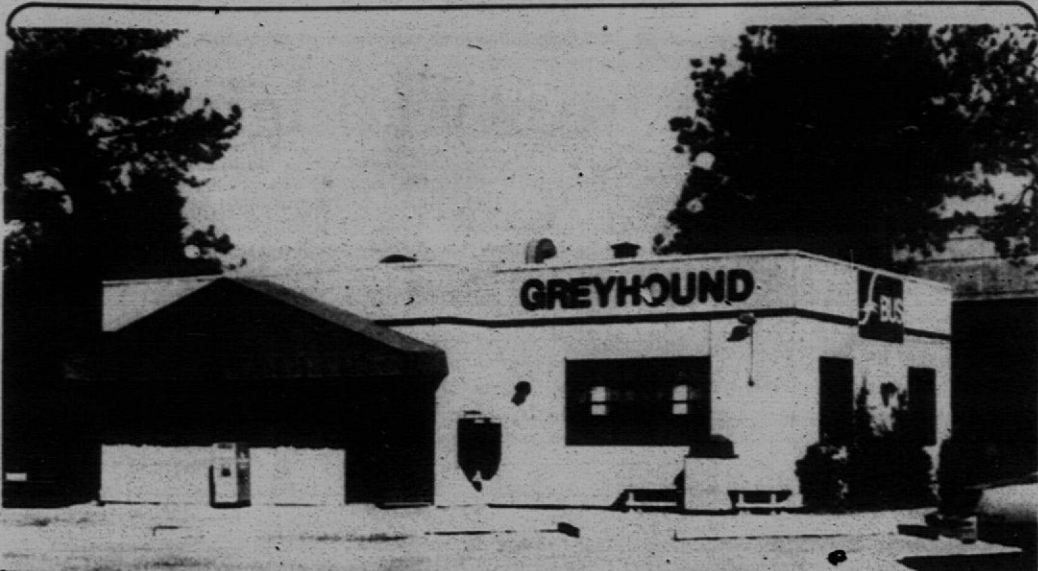
Bill Andrews The Greyhound Bus Terminal has been moved to 1351 Richmond Road, former site of the Hickory House Barbecue Pit Restaurant. Branches of Hertz Car Rental Agency and Western Union are also located in the refurbished building.
