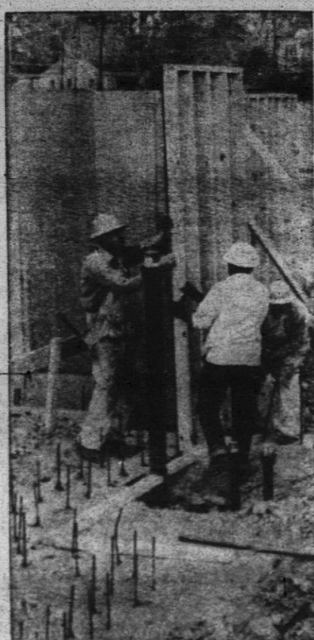
Crest carpenters install panels.
