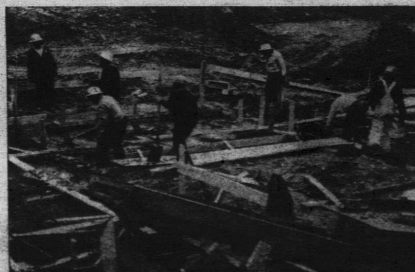
Under careful supervision workmen assist in pouring of concrete.
