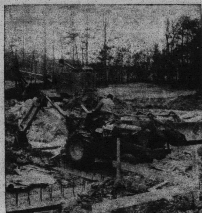
Final excavations are made prior to foundation work.
