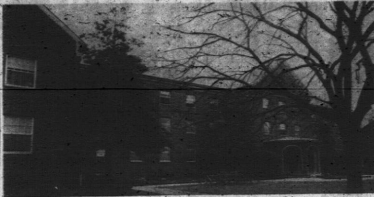
Dillard Complex was one of the many areas without heat after break.
