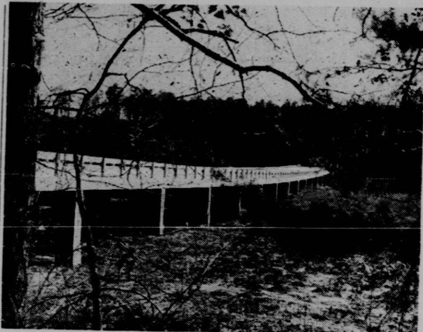
Half Way Creek Bridge, located three miles south of Williamsburg. This bridge is to be tied into the Colonial National Monument Parkway.
