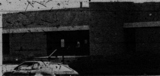
The Williamsburg Public Library is on Scotland Street.
