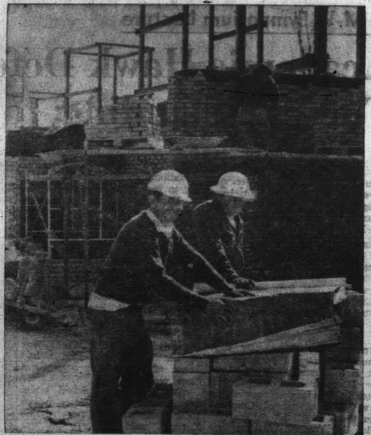
CONSTRUCTORS SCAN HOUSING BLUEPRINTS Several foremen examine the details depicted in blueprints of the new fraternity housing complex which is nearing completion on the new campus. Occupation of the tiered structures is planned for September of 1967. Photo by Randy Hawthorne.
