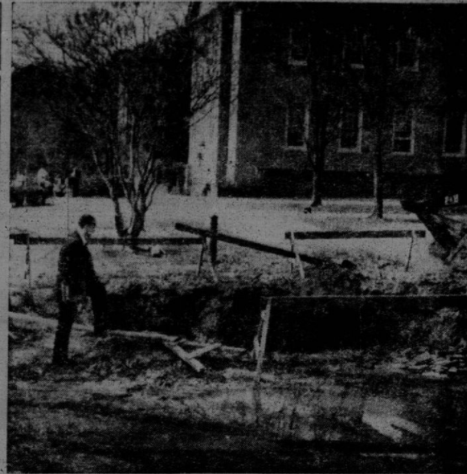
SPRING IS HOLE DIGGING TIME
