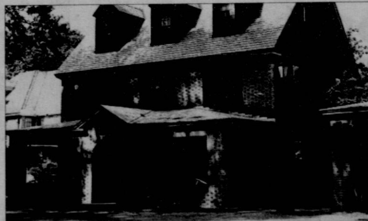
Security houses, Brown Hall and the Dillard complex have 24-hour security systems.
