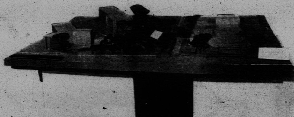
Construction of the Museum of Art will begin in late October. The building will be located between Morton and Phi Beta Kappa Memorial Halls.
